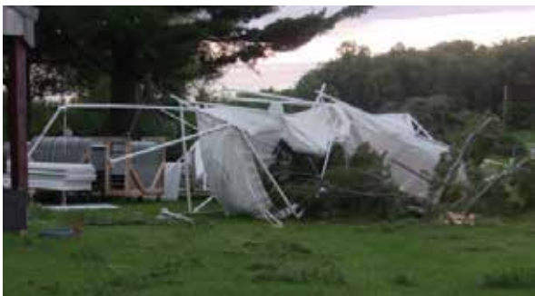
Damage was so extensive that cleanup will continue into 2020.
